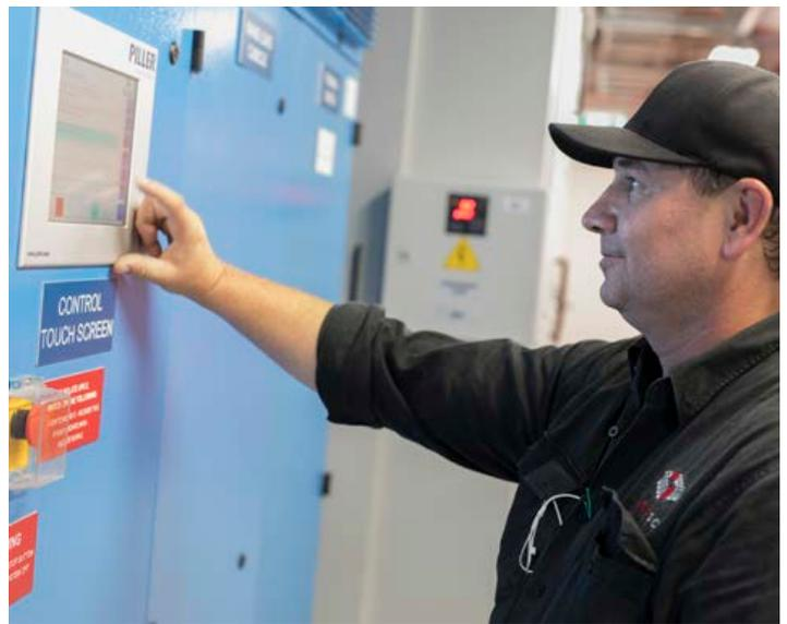
Above: The Piller Rotary UPS can support 1.6MW of load for up to 15 seconds while the MTU generator fires up.
