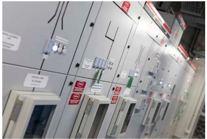
Above: ABB supplied boards enable Piller's Isolated-Parallel Bus-based electrical distribution and protection scheme (IP-Bus).
