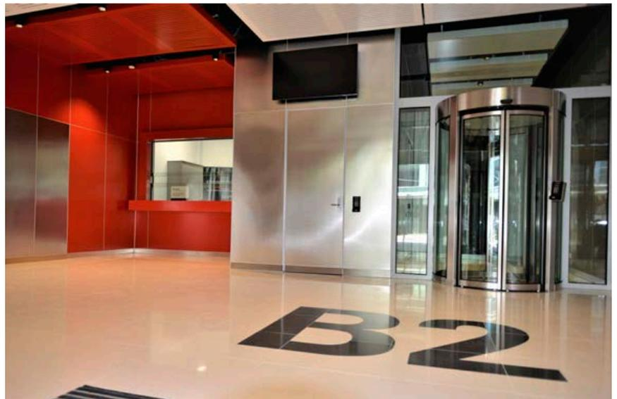
Above: Bullet-resistant security portals from Gunnebo provide access to the most secure areas, accessed via combined biometric fingerprint readers and swipe card authentication.
