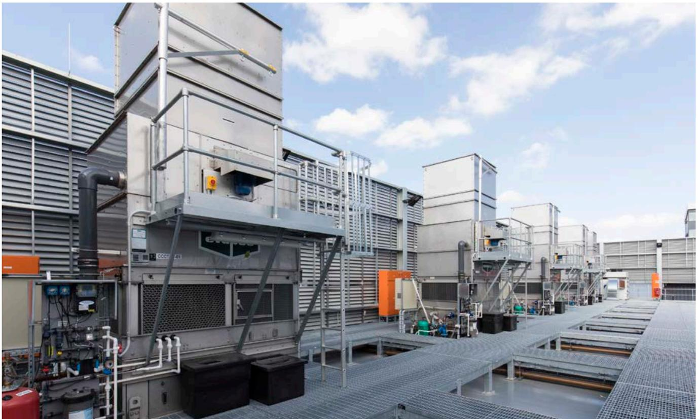
Above: B2 features incredibly efficient, stand-alone modular cooling tower units, instead of one large, central water plant unit, each linked to a different set of risers.
