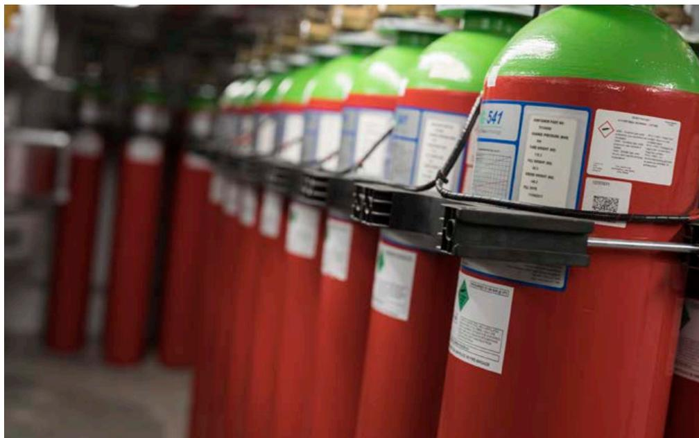
Above: Cylinders of inert gas for the fire suppression system.
